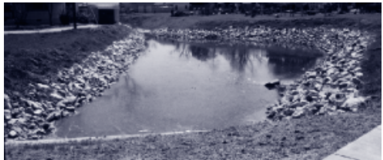
A well-kept retention pond with rip rap.
