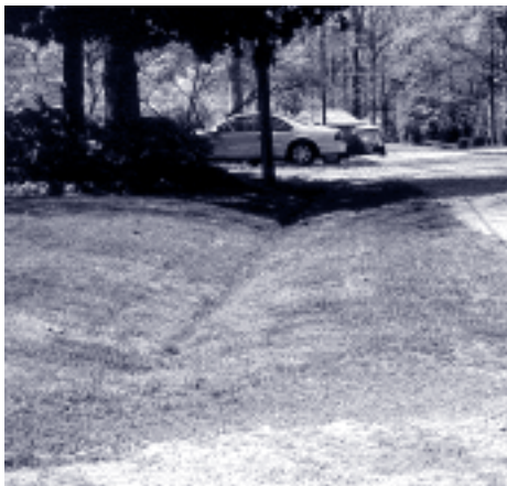
If you have a grassed swale like this in your yard, you have a BMP.
