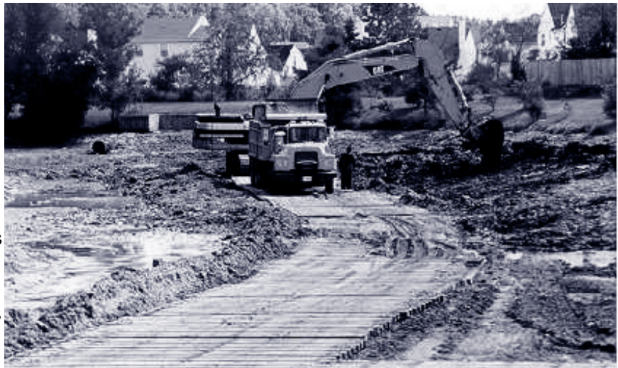
Dredging helps lower nutrient concentrations in water.
