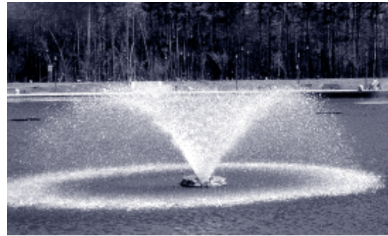
Aerators can be functional and decorative, unlike fountains which are only decorative.
