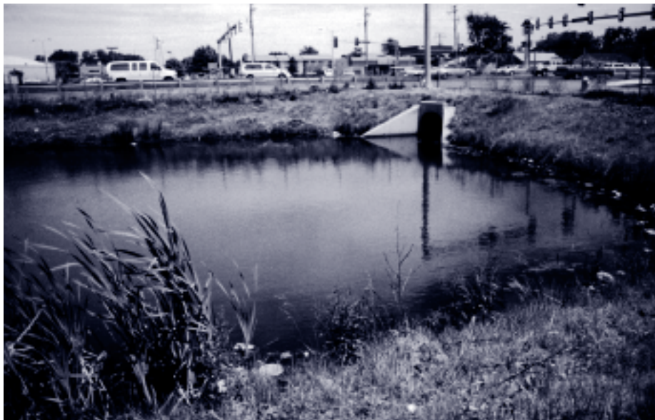
A properly functioning retention pond.
